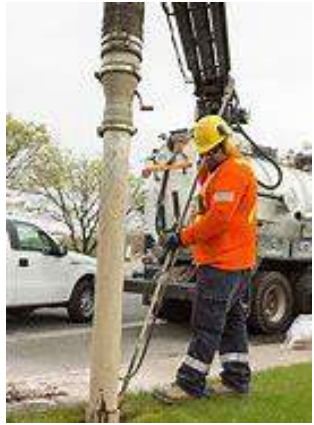
Catch Basin Inspection and Cleaning
